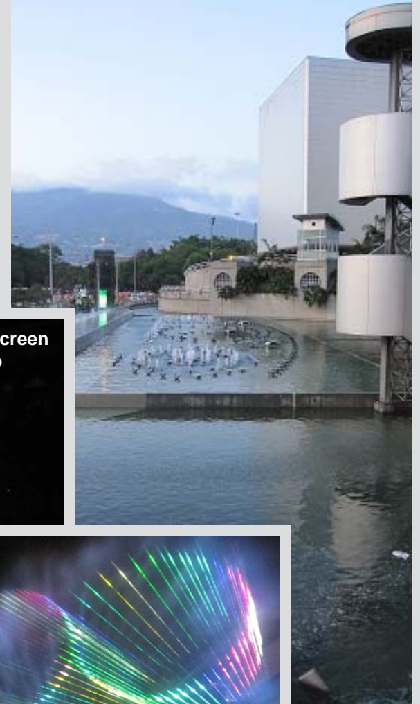
EPM Building Fountain
